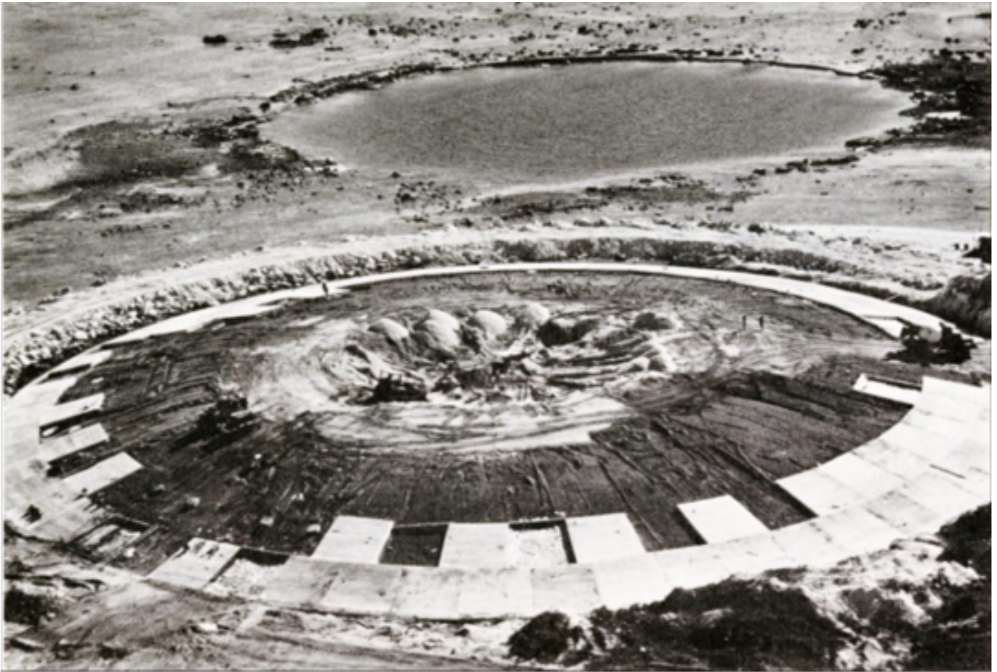
Concrete dome being poured on Runit, 1980
